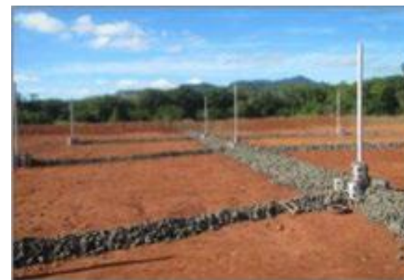
Key components of Fukuoka method – leachate collection and vertical gas venting pipes (Source: JICA/SPREP)
